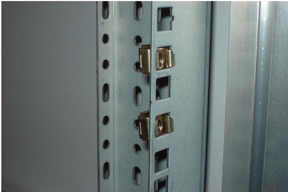
Figure 3-1. Fit cage nuts (not supplied).
