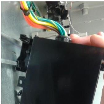
4. Snap the Isolation Module on the DIN rail. Alternately, the Isolation Module can be mounted to any surface using three, #8 pan head screws or another compatible fastener. Surface mounting with screws is recommended for high-vibration environments.
