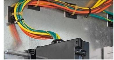
8. Route Sensor Leads and AVT System Cable to avoid sharp edges, pinch points and prevent mechanical damage.
