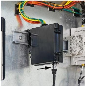
6. Insert the other end of the AVT System Cable in the connector on the bottom of the Isolation Module.
