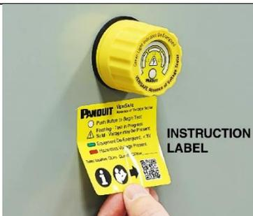
9. Install Instruction Label directly under or next to the Indicator Module on the exterior of the enclosure (see Note 1). Mark the label to indicate where in the circuit the AVT is installed.
