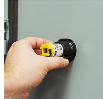
3. Tighten the panel nut until both it and the sealing washer make full contact with the enclosure surface. Then, tighten an additional ¼ turn. Tighten the panel nut with fingers only, do not overtighten.
