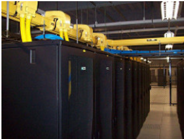
Figure 21 FiberRunner® Cable Routing System Installation
