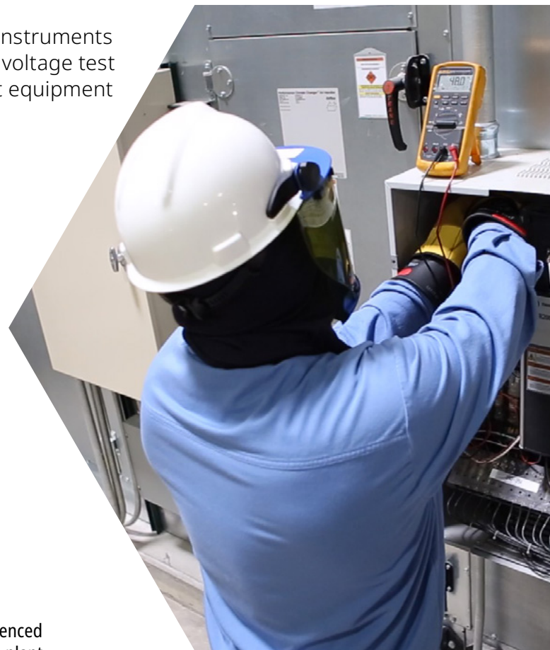
Figure 1: Absence of voltage test using a hand-held voltage test instrument.
